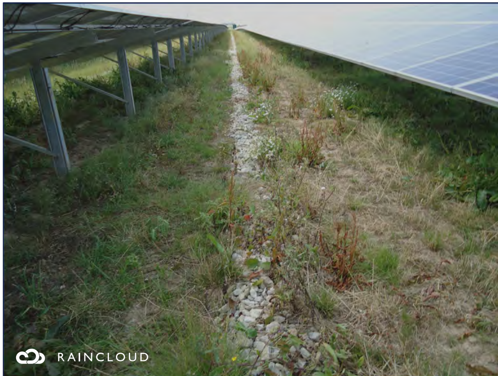
Plate A9.1.20: Example filter drains at solar farms
